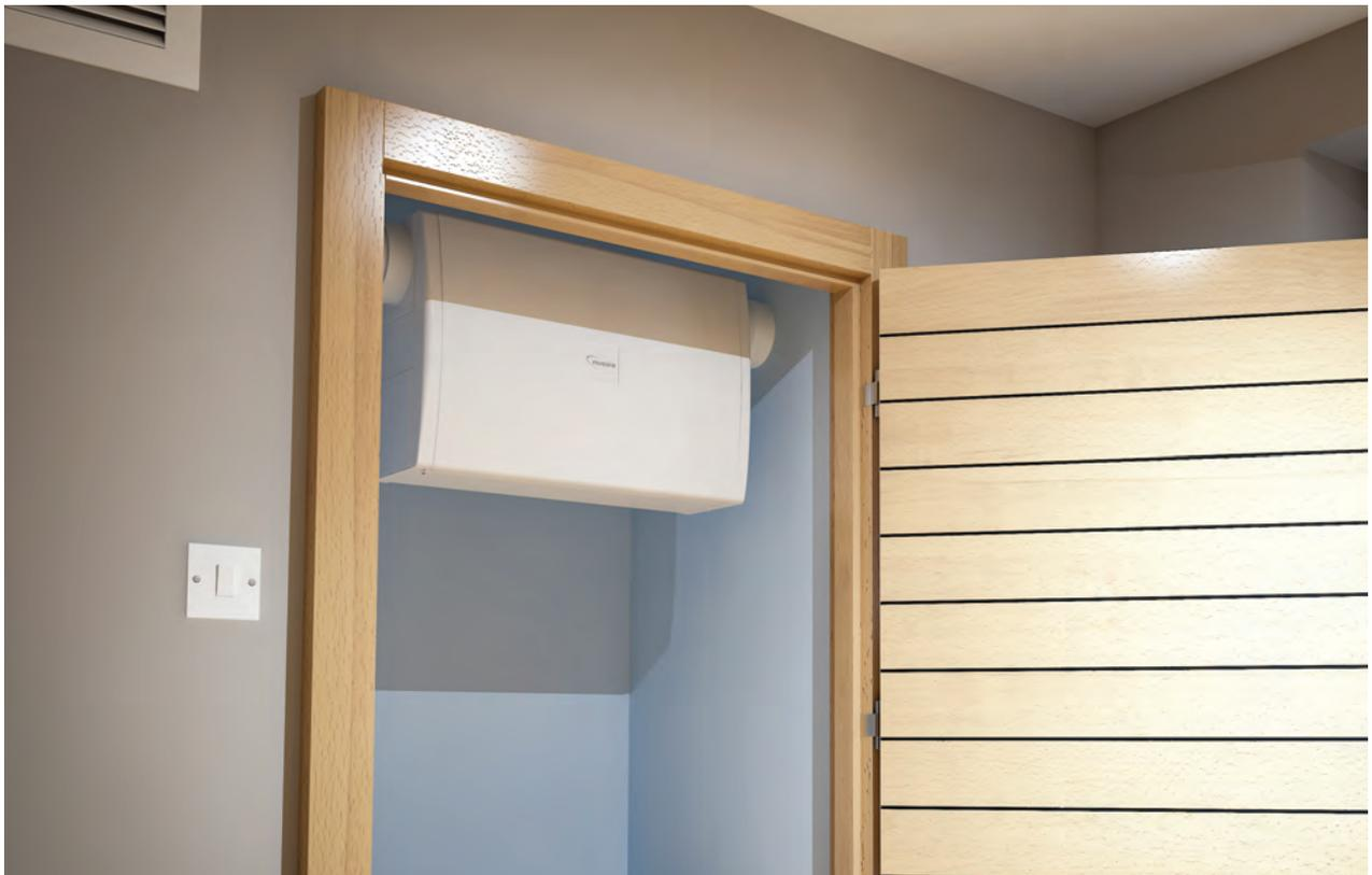
PIV systems are proven to be effective units in significantly reducing radon gas levels in affected areas.
